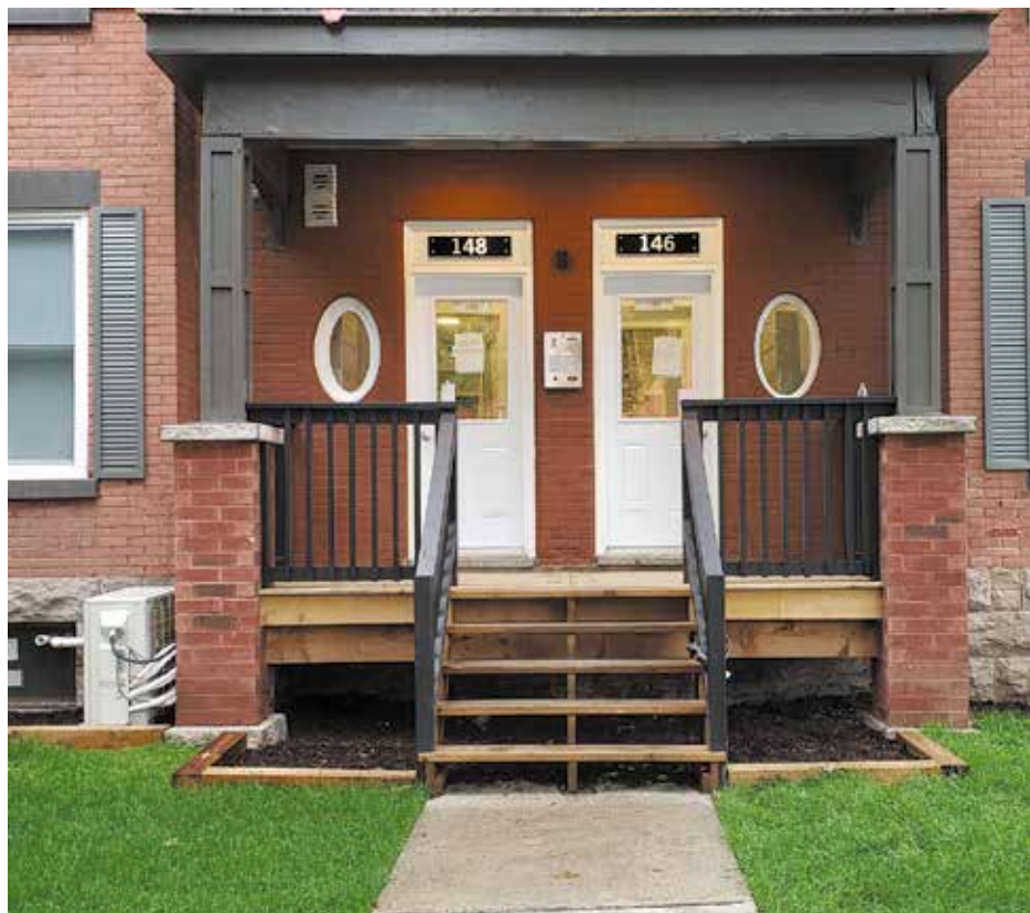
146 Osgoode after renovation.
