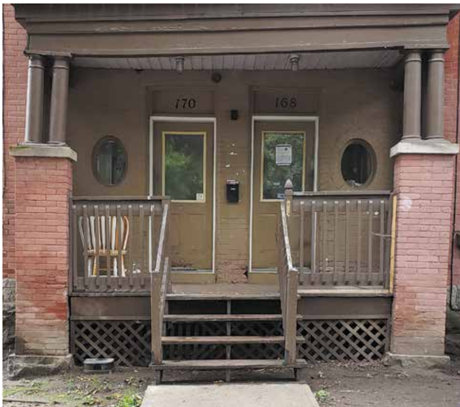
168-170 Osgoode before renovation.
