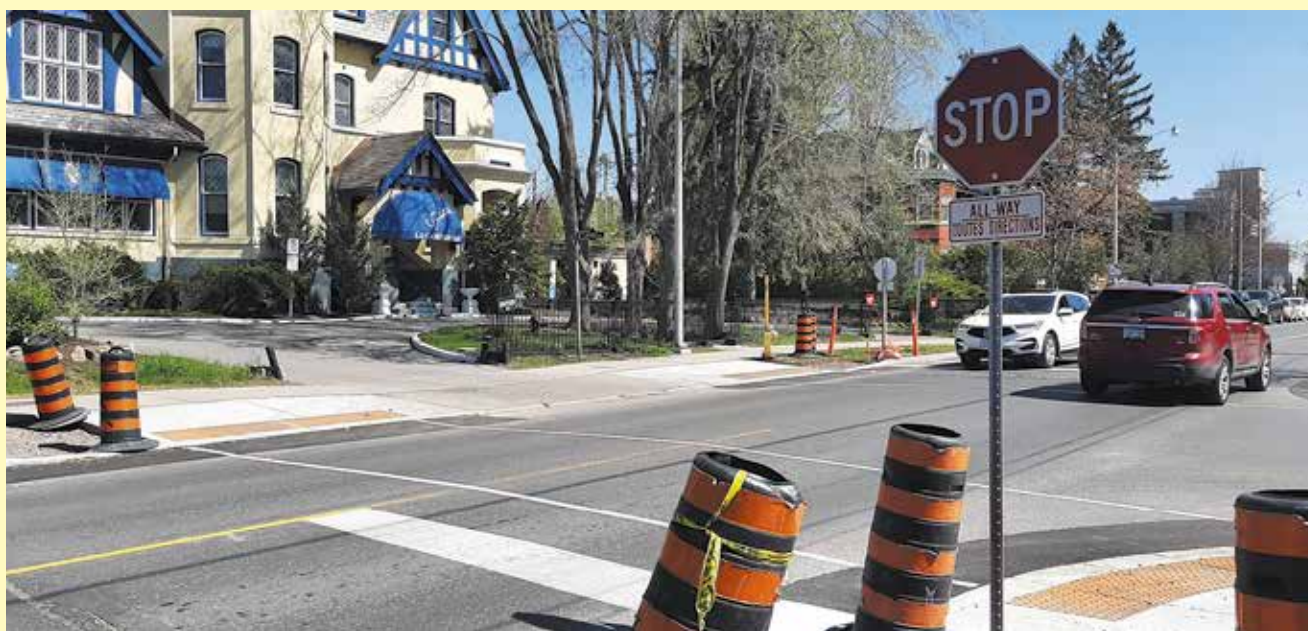
Above — During mid-May major intersection work at the corner of Range Road and Laurier Avenue was completed to include a three-way stop and pedestrian calming extensions to the curbs along with new street markings. The remedial work at this intersection will greatly improve pedestrian and vehicle safety at this busy intersection.
