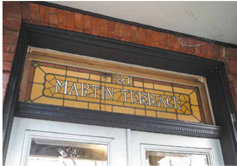
The recently remounted window at 521 King Edward Ave. While each of the four properties has a stained glass window above the front entranceway, this was the only one that included the original name of the property.
