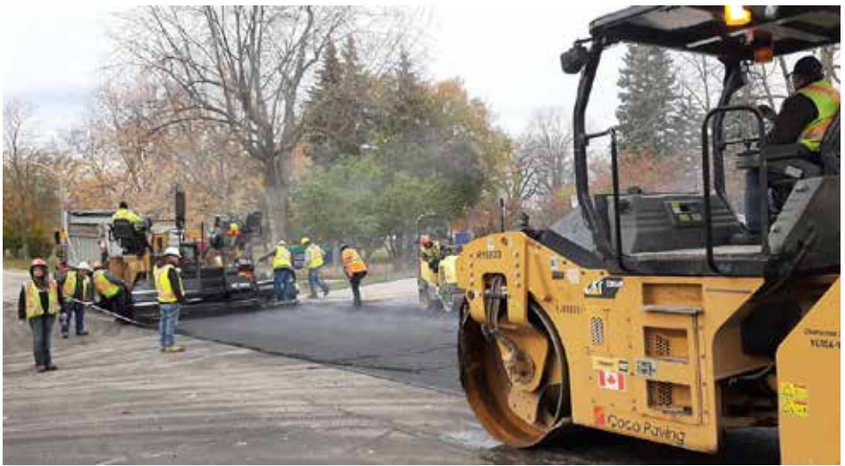
Oct. 28— the final load of pavement is rolled into place at the corner of Somerset and Range Rd. Water and sewer services are replaced after a year of traffic disruption.
