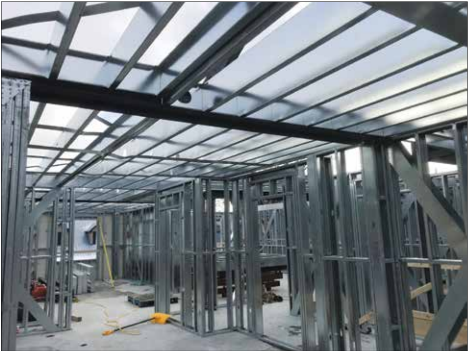
Factory fabrication work means that the frames are ready to be assembled at the building location complete with predetermined and pre-drilled junction points.
