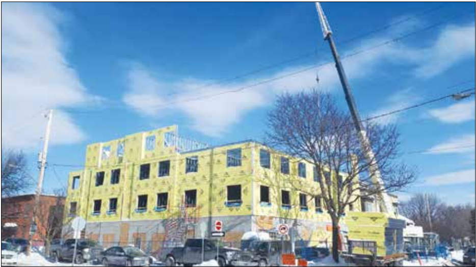
An on-site crane places the pre-assembled panels in place as the building takes shape.
