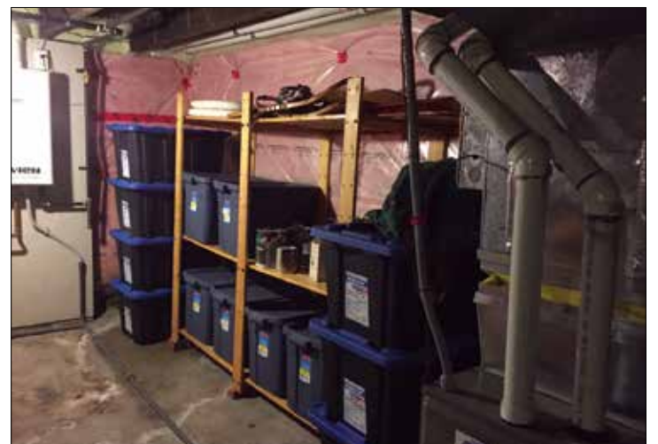
Tankless hot water on left, high efficiency furnace on right.
