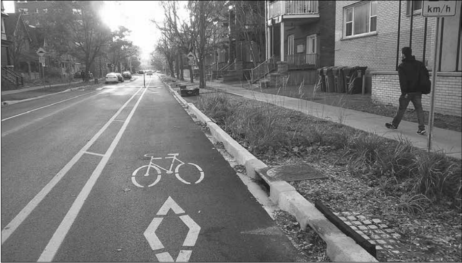
This photo shows the opening in the newly moved and reconstructed curb where the water drains off the street and into the new wider green area with added plants between the curb line and the sidewalk. This configuration is on both sides of the street.
