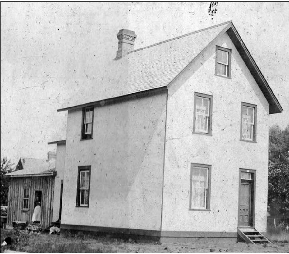
The original stucco-covered structure had no foundation at all.
