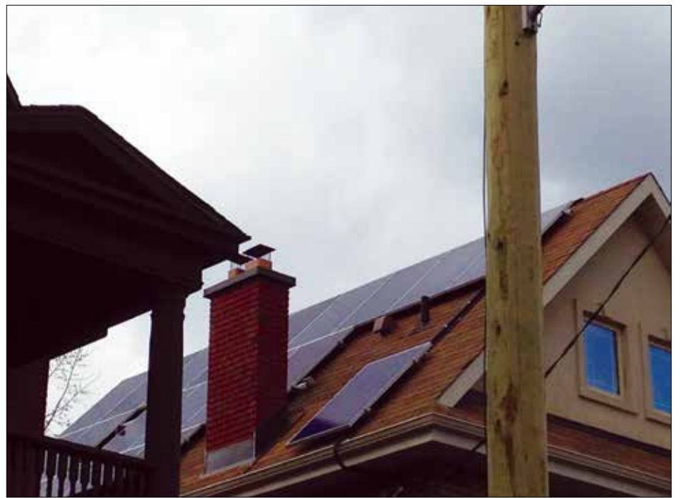
Solar panels on a neighbourhood roof feed electricity into the provincial grid. After two panels failed, a wire-mesh skirt was added around them to protect the soy-based coating on the wires from those well-known voracious, high-climbing Sandy Hill squirrels.
