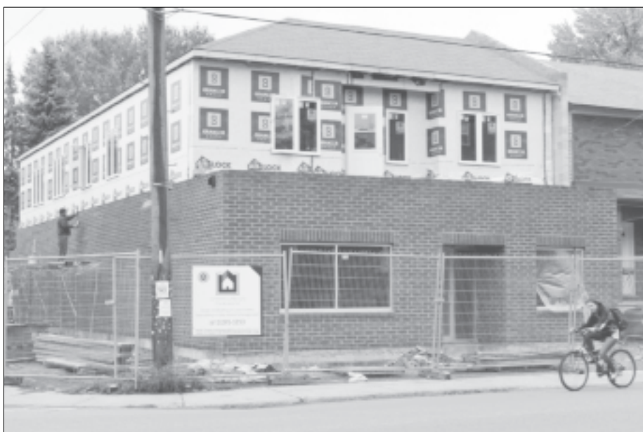
The new Ayoub's at Blackburn and Somerset East looks much the same as pre-fire.
