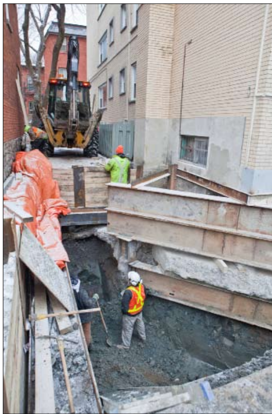
These foundation repairs at Stewart and Nelson Streets in January got going before the firm in charge applied for a building permit. Neighbours beware: these things can happen! Photo Bill Blackstone
