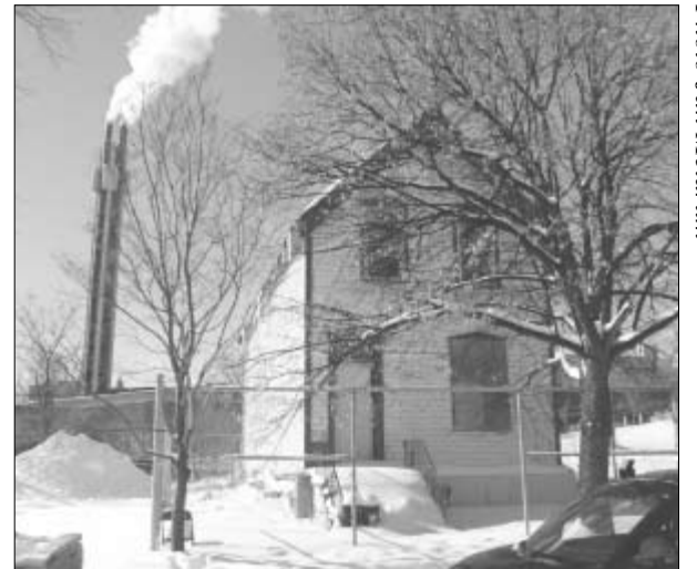
Derelict house, 206 Henderson Ave., owned by the University of Ottawa; its demolition is pending city approval.
